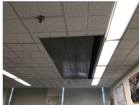
Chemistry Classroom Unit Ventilator
