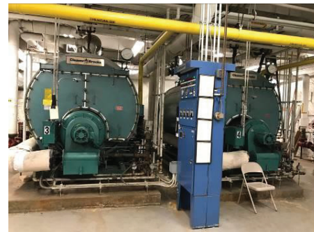
Existing Boilers, B-3 & B-4
