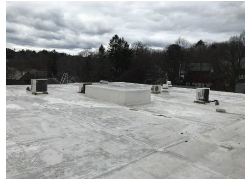
Ductless Split System Condensing Units
