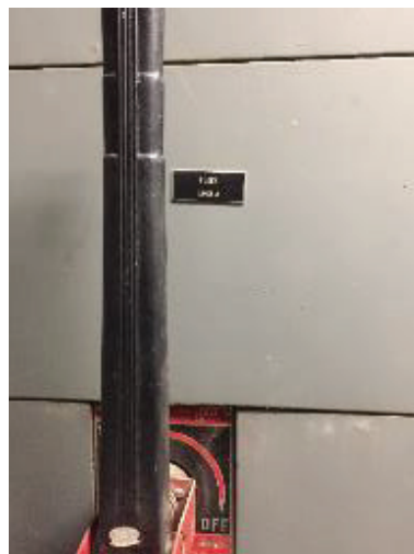
Original Vintage Main Fuse Switch
