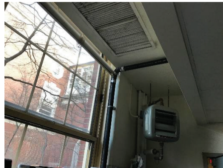
Restaurant Kitchen Supply diffuser and Unit Heater
