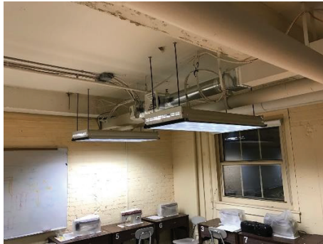
Basement Classroom Exhaust Fan
