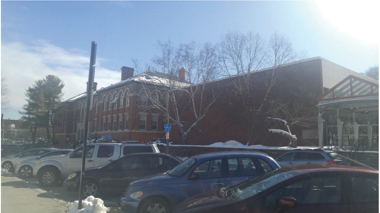
Looking south at the gymnasium along Tappan Street
