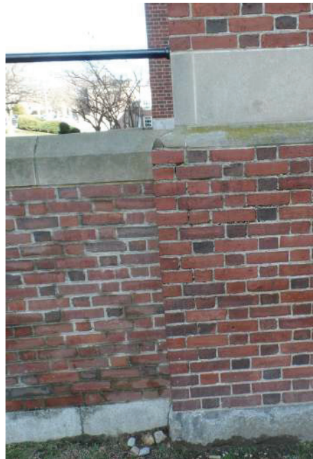
Photo 18: Moisture Damage at Site Wall and Building Wall - Main Campus
