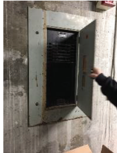
Existing Original Vintage Panelboard
