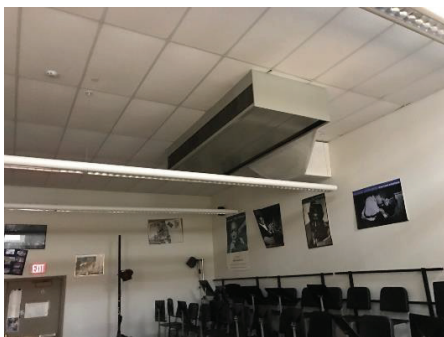
Music Room – Ceiling Unit Ventilator
