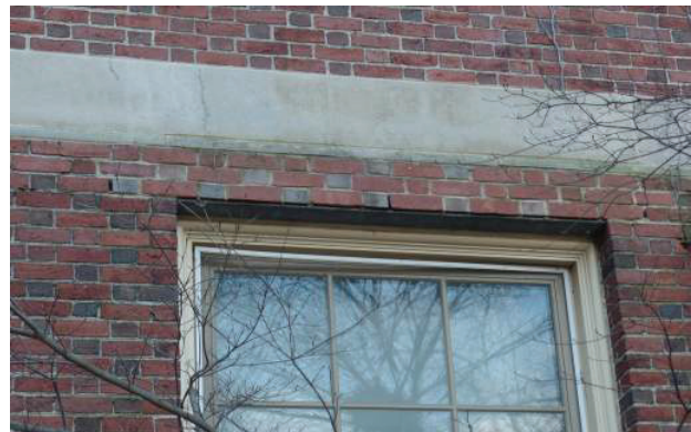
Photo 6: Rusting Lintels - Main Campus
