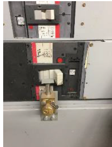
800 AMP Breaker for Temp. Generator
