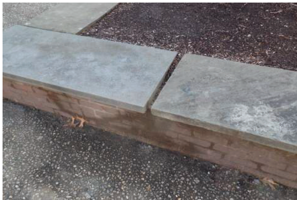
Photo 5: Open Site Wall Cap Stones - Main Campus Courtyard
