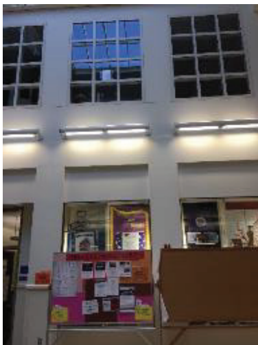
Main Lobby Lighting
