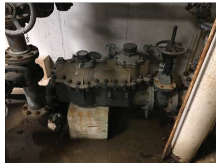
Domestic water meter
