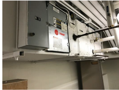
Basement Air Handling Unit
