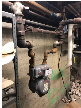
Interior gas meter
