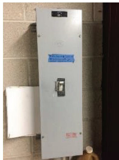
Breaker for Manual Transfer Switch
