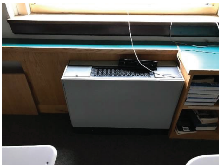
Classroom – Hot water Cabinet Unit heater
