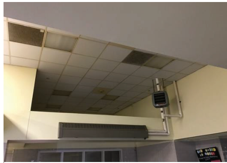
Wall mounted Fintube radiation and Unit Heater
