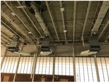
Third Floor Gym – H&V Units
