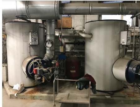
Gas-fired domestic water heaters
