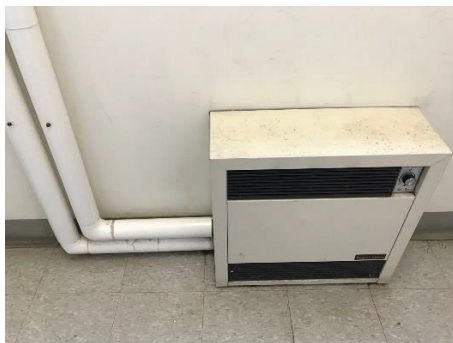
UAB Corridor Cabinet Unit Heater
