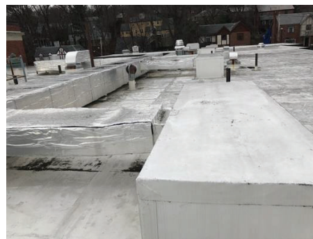
Roof mounted insulated ductwork
