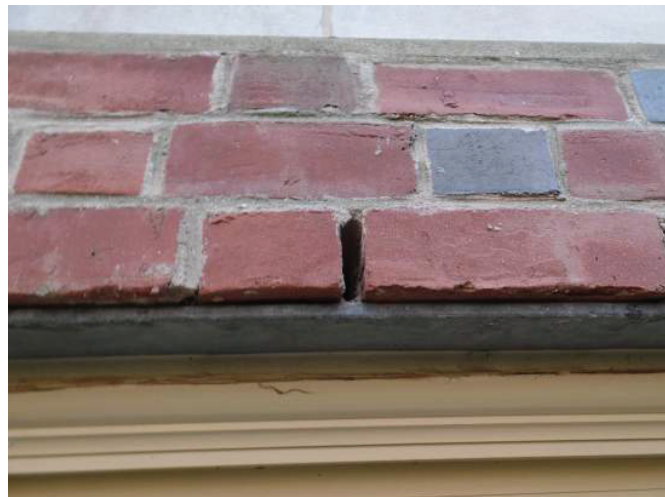
Photo 16: Galvanized Steel Replacement Lintel (with Weep Hole) and New Window - Main Campus
