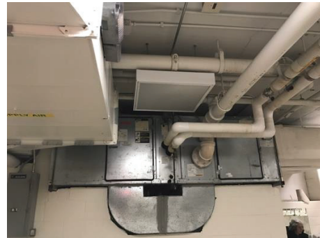
Locker Room AHU
