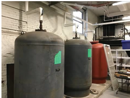
Hot Water Expansion Tanks
