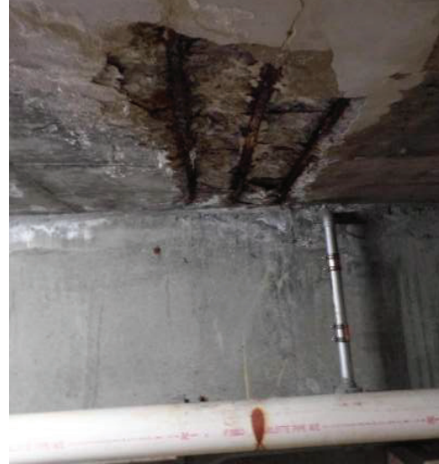
Photo 2: Deterioration in Pool Deck Slab at Former Diving Board Location
