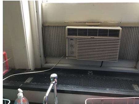
Classroom – Window AC Unit
