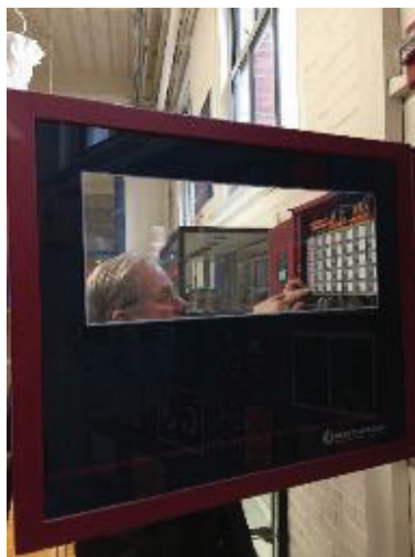
Fire Alarm Control Panel
