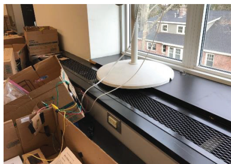
Fin tube Radiation in Enclosure
