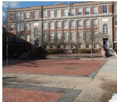
Photo 4: Cracks in Concrete Pavement - Main Campus Courtyard
