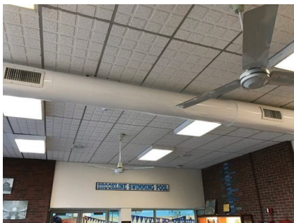
Pool Lobby Ductwork
