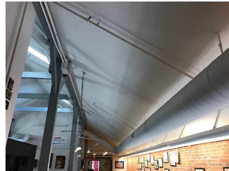
UAB Gallery – Exposed Ductwork
