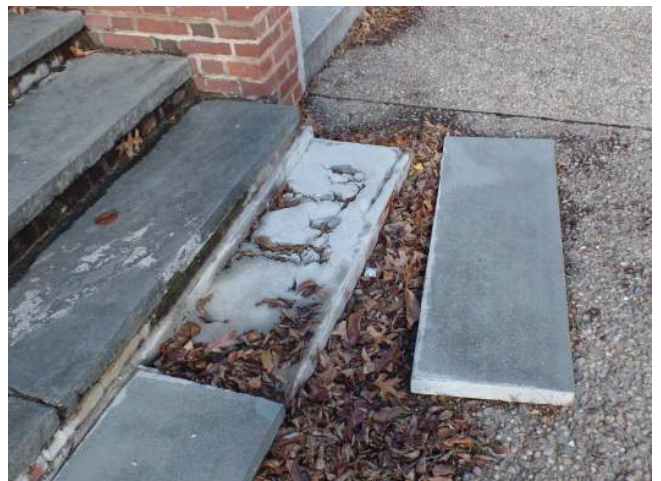
Photo 12: Deteriorating Site Stair - Main Campus
