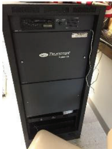
Classroom Intercom System Headend
