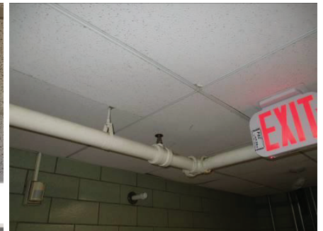
Upright type sprinkler
