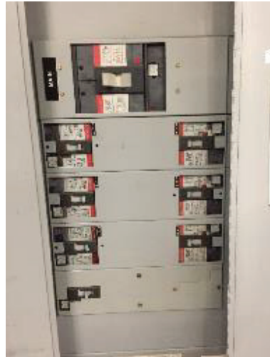
Central Plant Distribution Panel "CPNDP"
