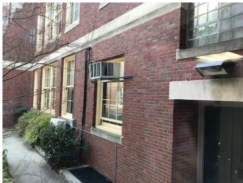
Window AC Unit and Grade mounted Ductless AC Condensing Unit
