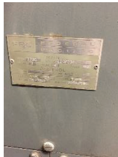
Original Vintage Main Switchboard
