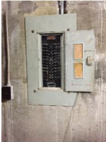
Existing Original Vintage Panelboard
