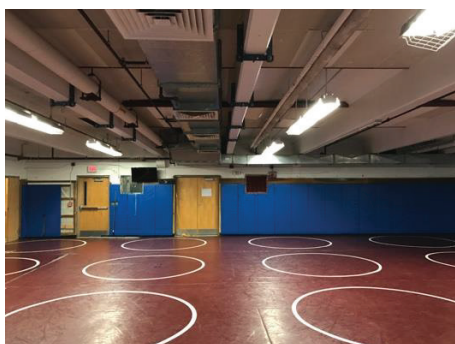
Wrestling Room-Ceiling Supply Ductwork
