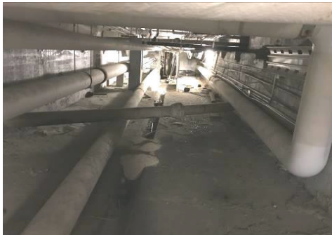
Main HS Building Tunnel – Hot Water Piping
