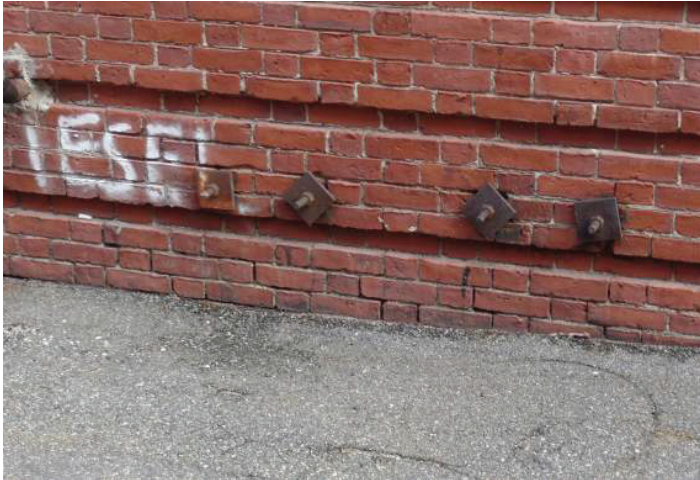
Photo 29: Repointing of Brick Veneer Needed at Base of West Exterior Wall - Unified Arts Building
