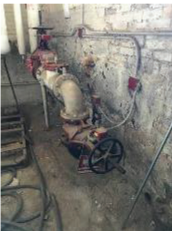
Fire service entrance
