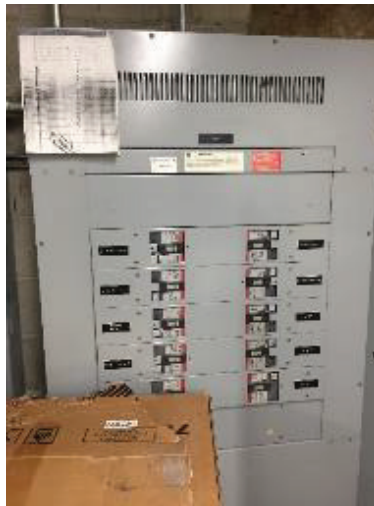
Typical Distribution Panel
