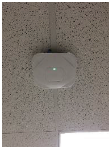
Wireless Access Point
