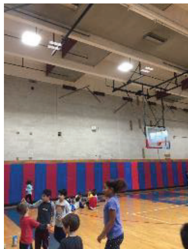
Broken Emergency Lights in Gym
