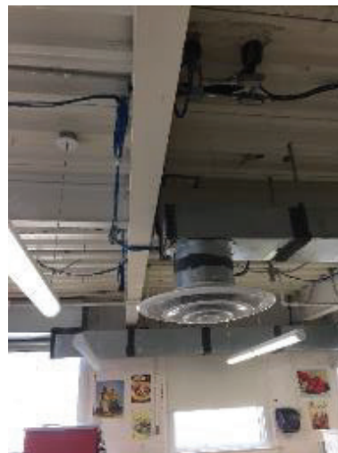
Exposed Data Cables
