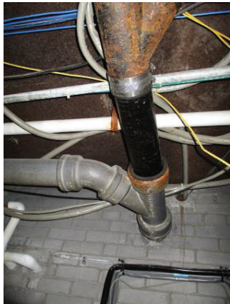
Cast iron drainage pipe
