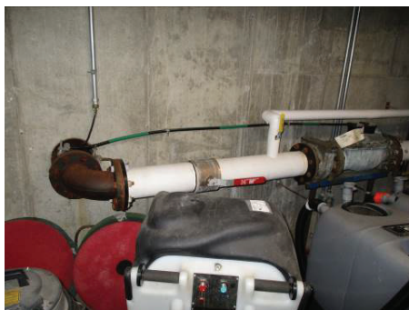
Domestic water service & meter
