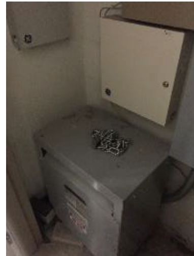
Other Equipment installed in 2-Hour Rated Life Safety Closet
