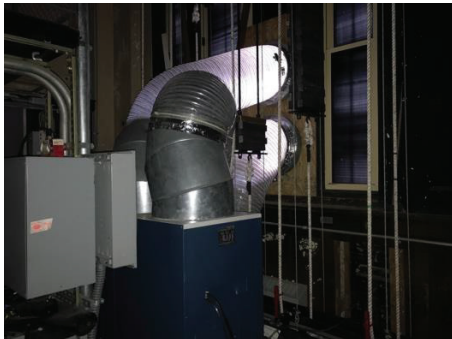
Stage – Portable AC unit
