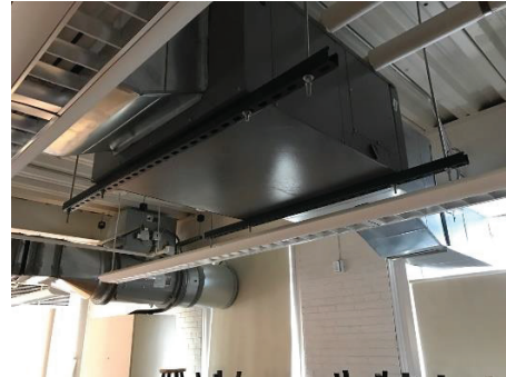
UAB Ceiling AHU unit and Exhaust Fan
