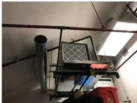
UAB Server Room – Split System AC Unit
