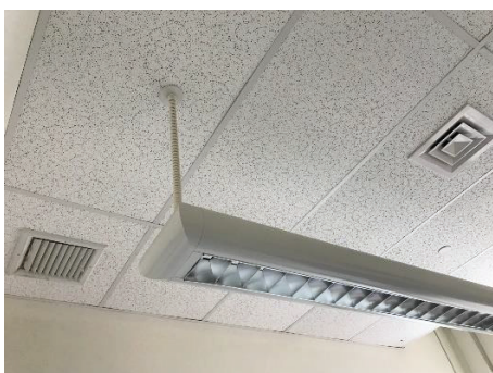
Office – Ceiling diffusers and registers
