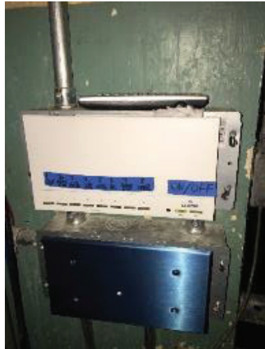
Theatrical Lighting Scene Controller
