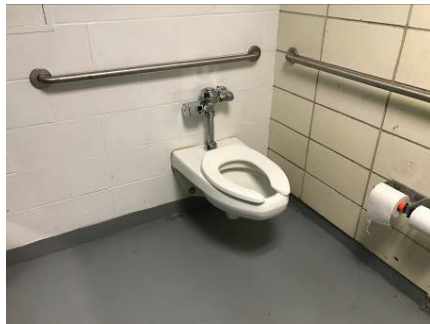
Wall hung water closet
