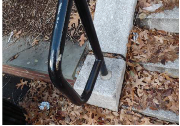
Photo 8: Open Cap Stone Joints at Site Stair - Main Campus
