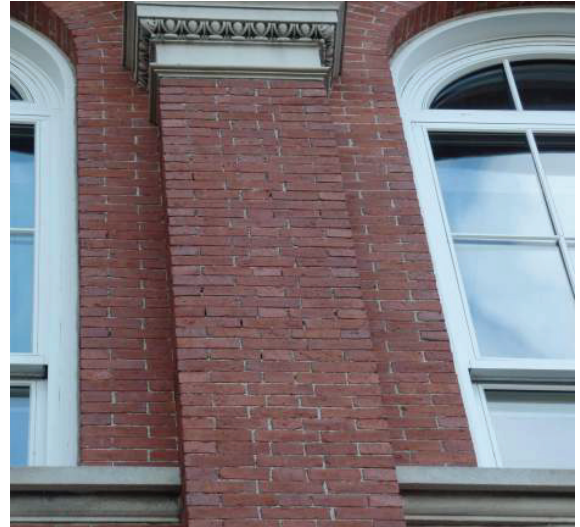
Photo 26: Repointing of Brick Veneer Needed - Unified Arts Building
