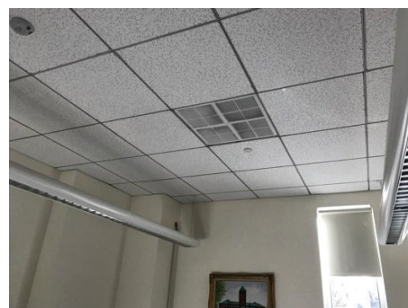
Office – Supply air diffuser
