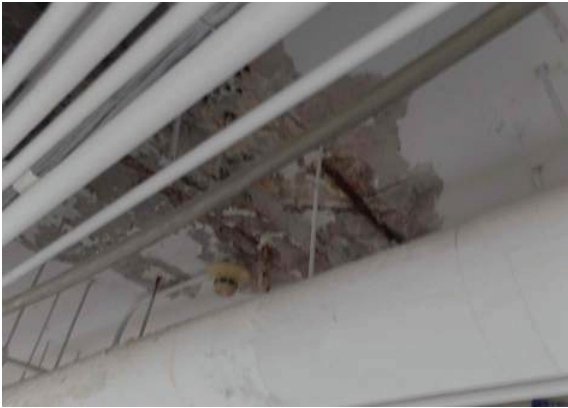
Photo 1: Deterioration in South Tunnel Roof
