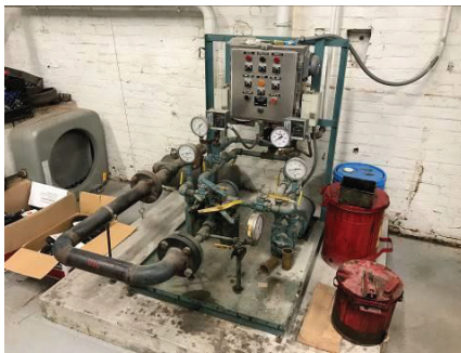
Fuel Oil Pumps
