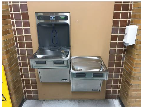
Hi-lo water cooler
