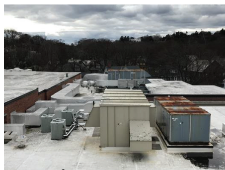
Auditorium – Rooftop Unit (center)
