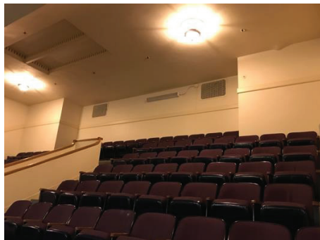
Auditorium- Sidewall Diffusers
