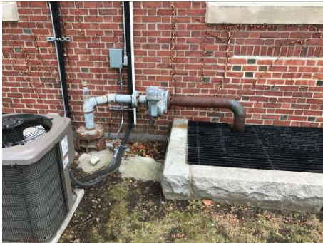
Exterior gas meter
