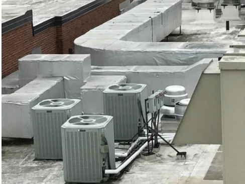
Roof mounted Air cooled Condensing Units
