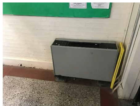
UAB Corridor Cabinet Unit Heater
