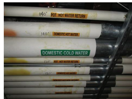
Domestic water piping
