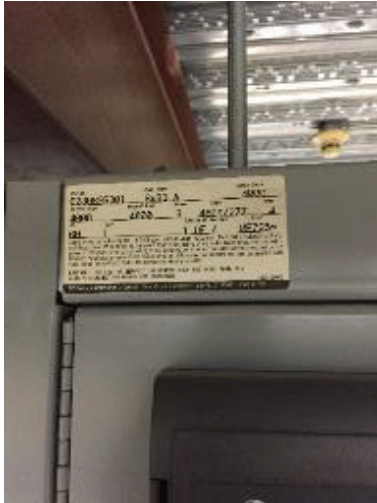
Main Switchboard Name Plate
