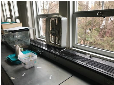
Classroom – Radiation Heating and Box Fan
