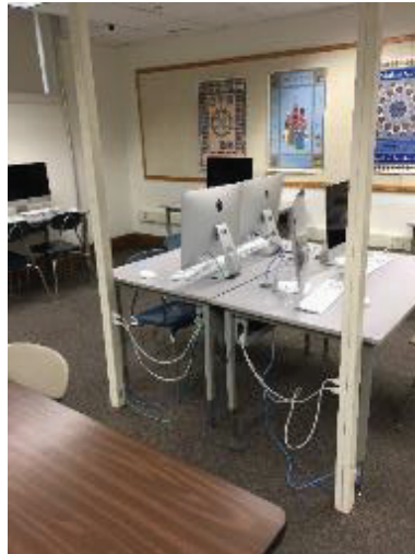
Power Poles in Mac Lab
