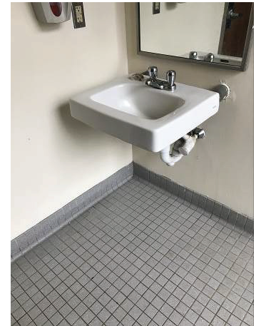
Wall hung lavatories
