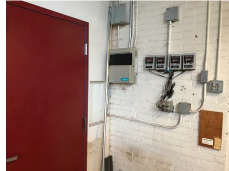
Unified Art Building DDC Control Panels
