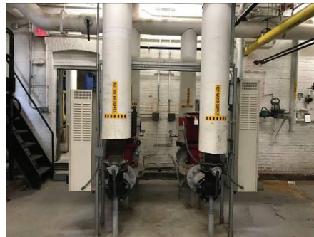
Primary Loop HW Pumps
