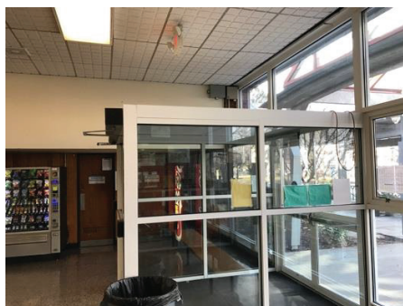
Pool Building Entry Vestibule
