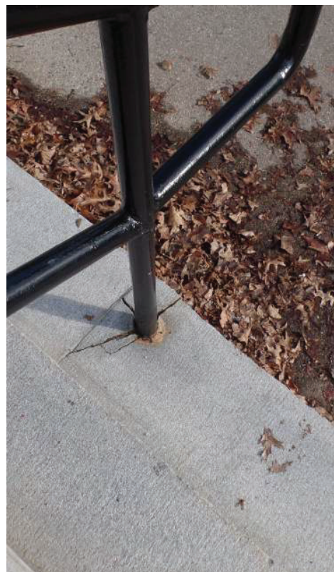
Photo 24: Concrete Damage at Entry Stair Railing - Tappan Gym
