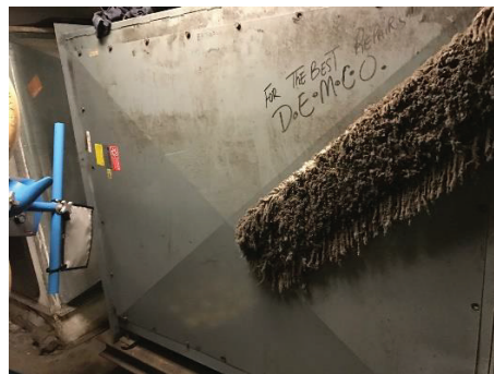
Third Floor – General Exhaust Fan
