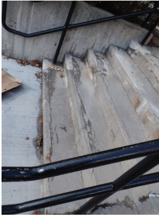
Photo 17: Deteriorating Site Stair - Main Campus
