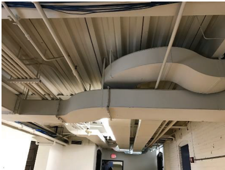
UAB Basement – Exposed Ductwork
