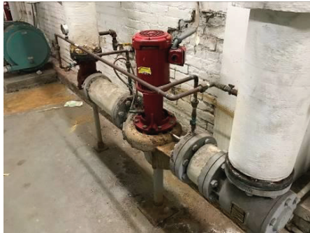
Primary Boiler Loop Circulator Pump
