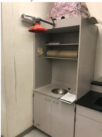
Science emergency fixture
