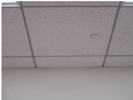
Concealed type sprinkler
