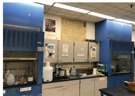
Prep Room - Fume Hoods
