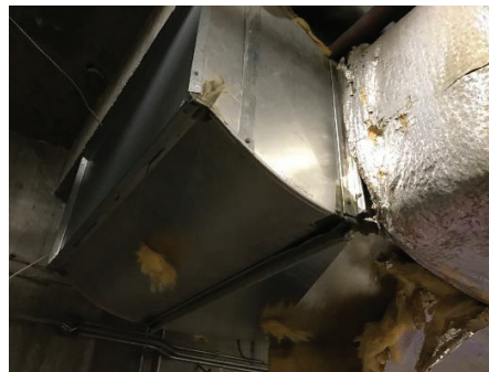
Pool Ductwork with missing insulation
