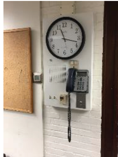
Classroom with VOIP Handset
