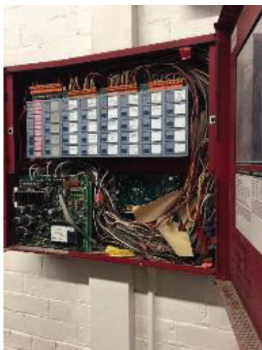
Fire Alarm Control Panel
