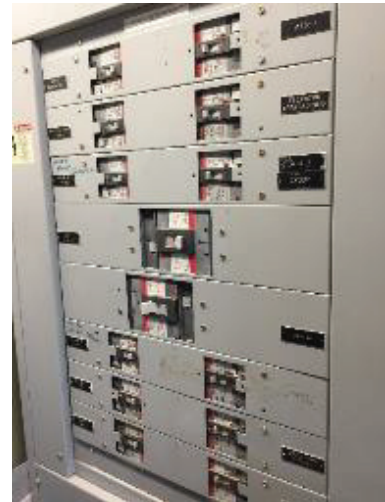
Switchboard "C" Distribution Section
