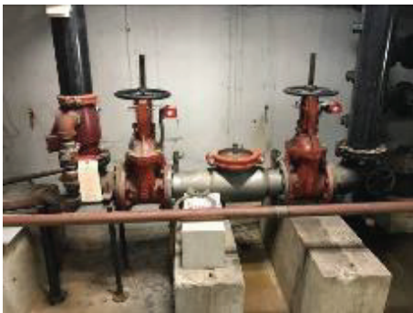
Double check valve assembly & alarm valve
