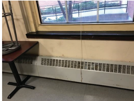
Cafeteria Overflow – Fintube Radiation
