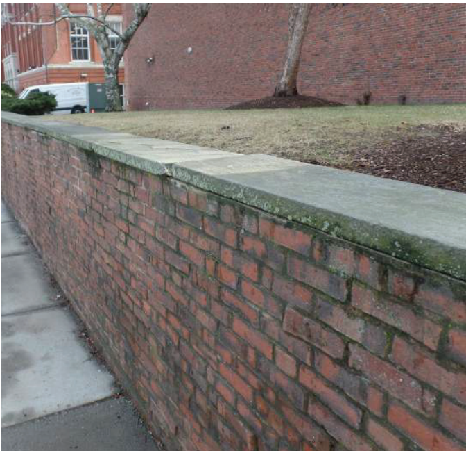
Photo 31: Moisture Damaged Brick and Loose Cap Stones - Tappan Gym/Pool Complex
