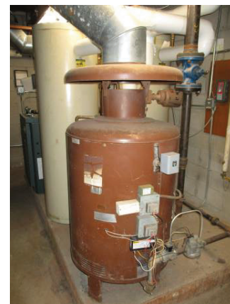
Domestic water heater #1
