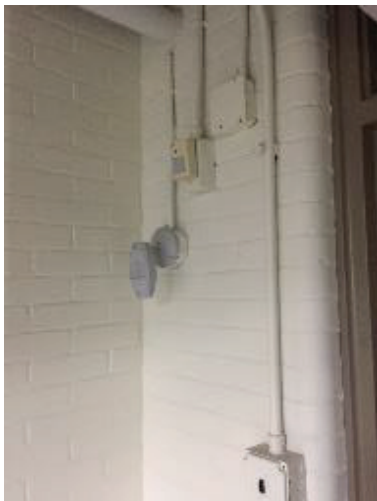
Motion Sensor in Corridor
