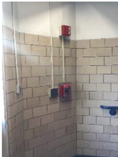
Typical Pull Station and Horn Strobe
