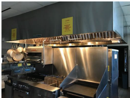
Restaurant Kitchen Exhaust Hood
