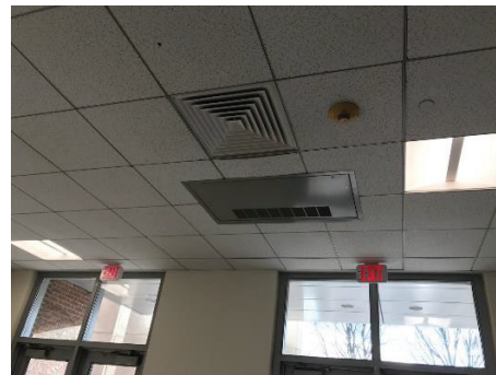
Main Entry – Ceiling Unit Heater
