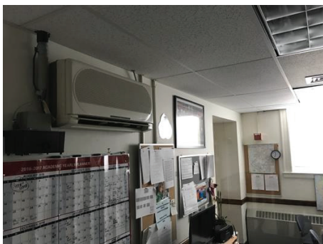
Office –Ductless AC Unit
