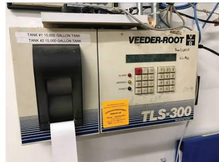
Fuel Oil Monitor Panel
