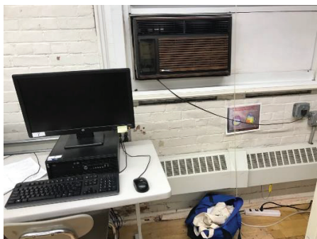
UAB Classroom – Window AC and Fintube Heating
