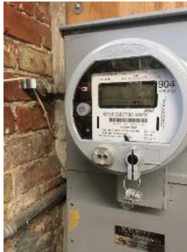
Unified Arts Utility Meter
