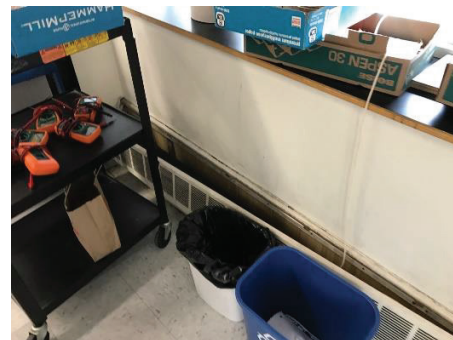
Classroom – damaged fin tube radiation enclosure
