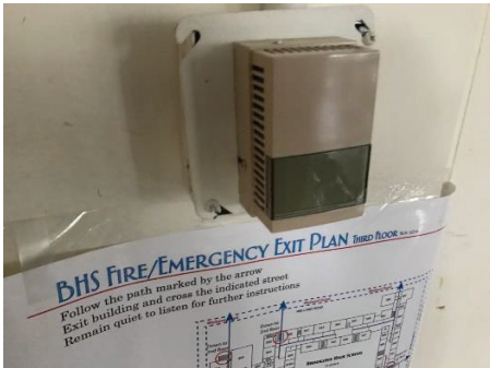
Newer Siemens Temperature Sensor
