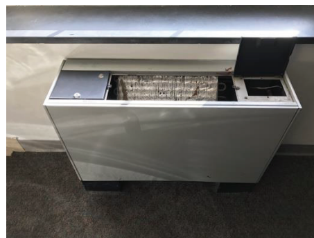
Phys. Ed. Classroom – Cabinet Unit Heater with Missing Grille
