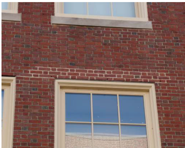
Photo 15: Lintel Replacement and New Windows - Main Campus
