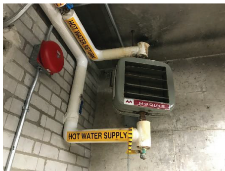
Basement Storage Room – Unit Heater
