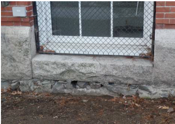
Photo 3: Exposed Rubble Stone Foundation at the Unified Arts Building
