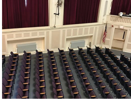
Auditorium – Hot water convectors
