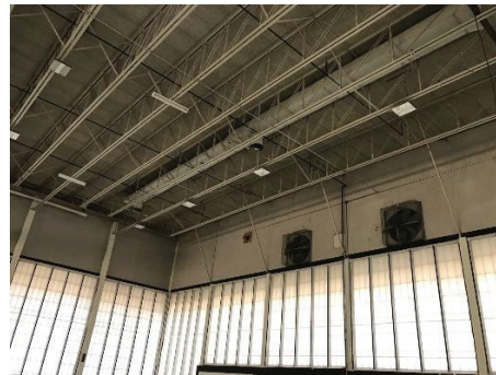
Third Floor Gym – Sidewall Exhaust Fans
