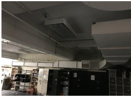
White Box – Exposed Ductwork
