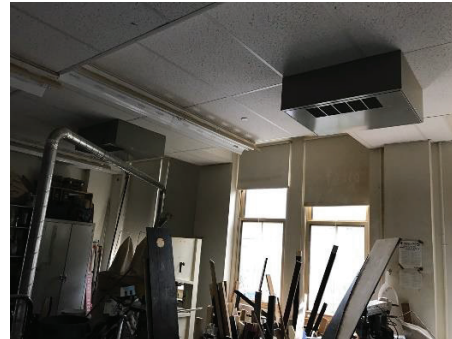
Scenery Shop Ceiling Unit Heater
