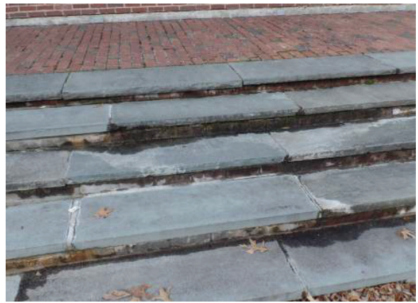
Photo 10: Deteriorating Site Stair - Main Campus
