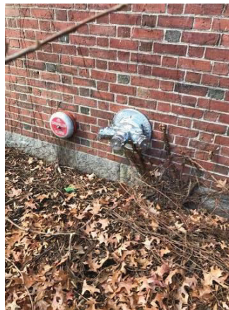
Fire Department Connection
