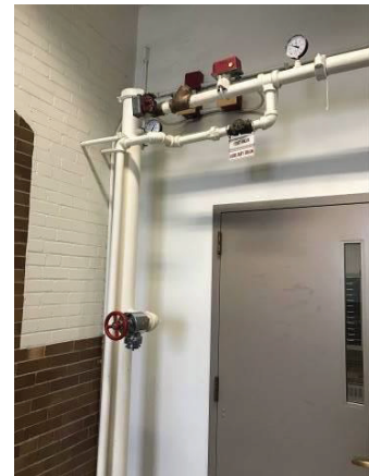
Typical sprinkler zone control valve
