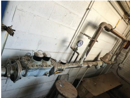
Domestic water service and meter
