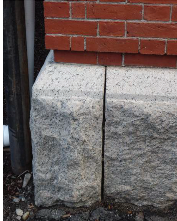
Photo 30: Open Joints in Stone Foundation - Unified Arts Building
