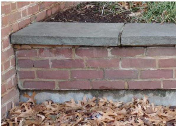
Photo 9: Deteriorating Site Wall - Main Campus
