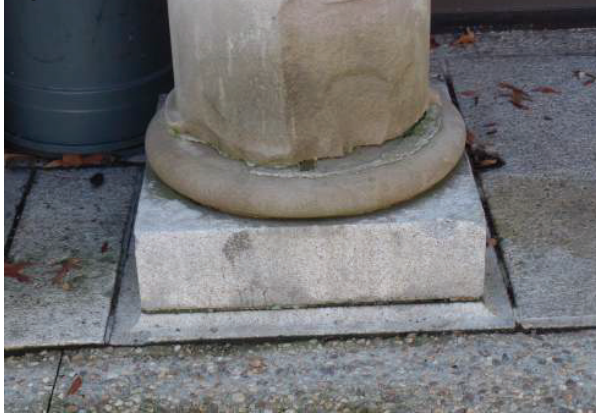
Photo 7: Deteriorating Column Base - Main Campus
