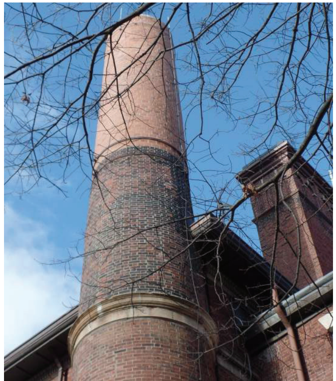
Photo 28: Repaired/Repointed Boiler Stack - Unified Arts Building
