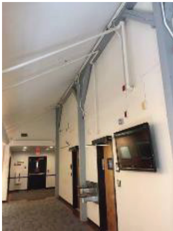
Typical exposed sprinkler piping and upright sprinkler heads
