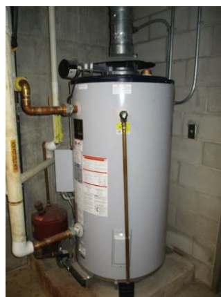
Non-potable water heater
