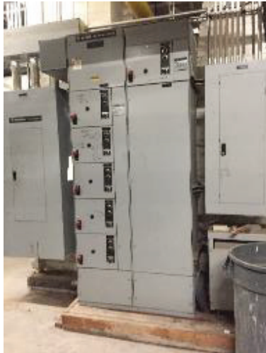
Central Plant MCC
