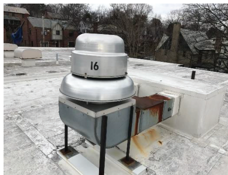
Roof Exhaust Fan with exterior ductwork
