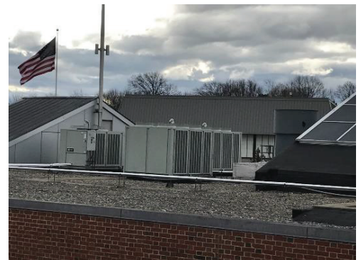
Rooftop Unit – Split Condensing Units
