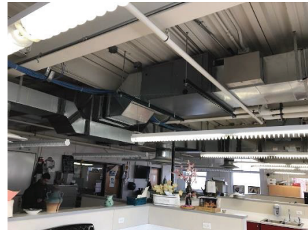
UAB Classroom – Ceiling AHU & Ductwork
