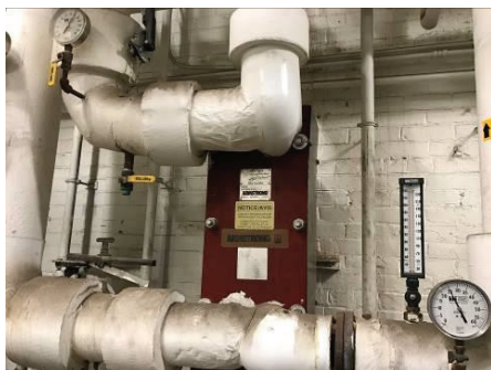
UAB - Plate & Frame Heat Exchanger
