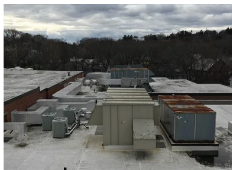
Rooftop Air Handling Units and Condensers
