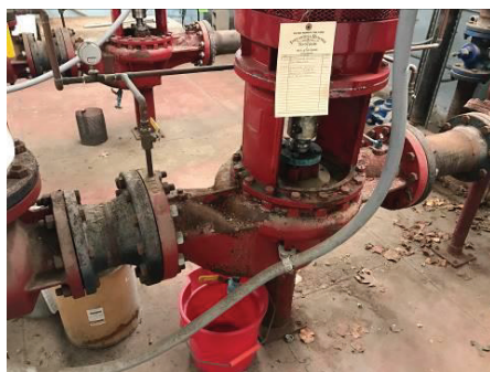
Hot Water Pumps
