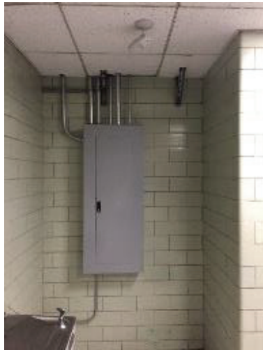
Typical Branch Circuit Panel Board
