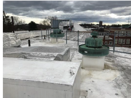
Older Roof Ventilators
