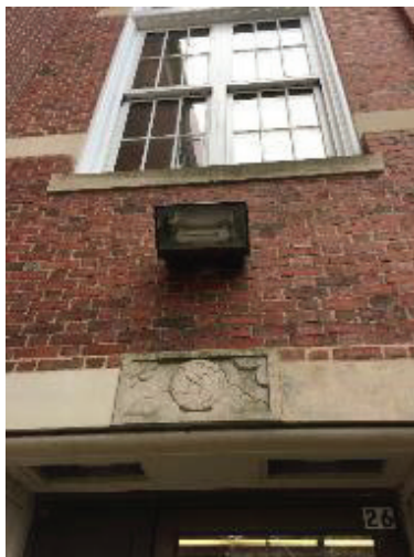
Induction Lamp in Exterior Wall Pack
