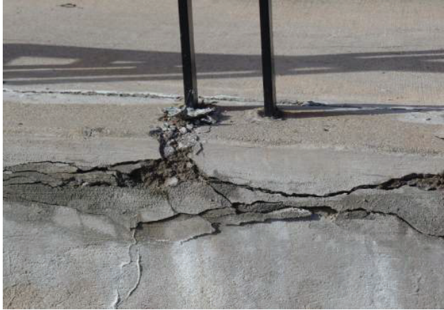
Photo 25: Concrete Damage at Entry Ramp Railing - Tappan Gym
