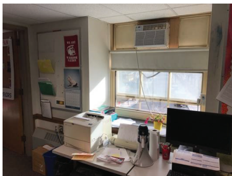
Athletic Dept Office – Window AC Unit
