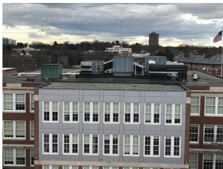
Rooftop Units (RTU-1,2&3)
