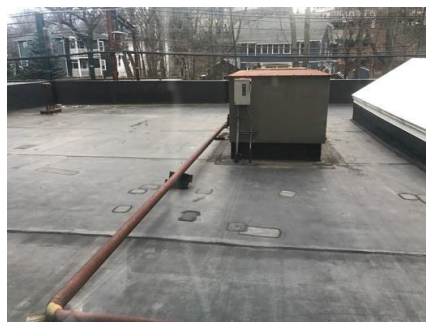
Boiler Room H&V Unit
