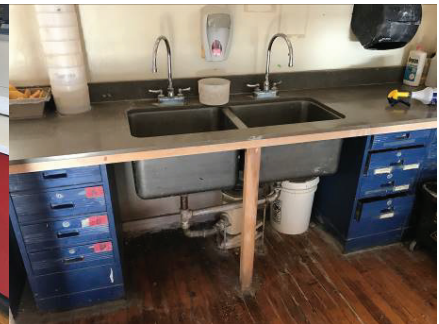
Art room sink with sediment trap
