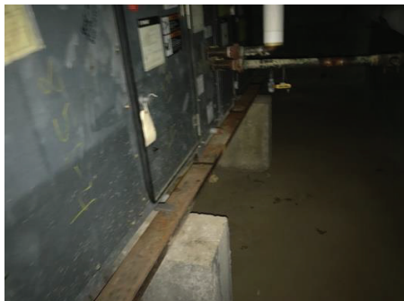
Pool Basement – AHU – Missing HW Piping Insulation
