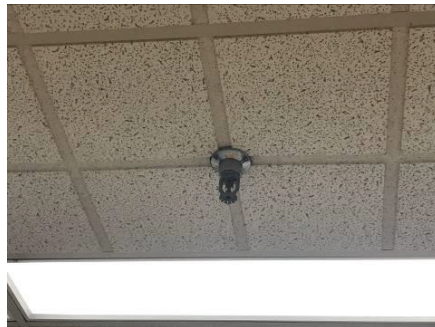
Pendent type sprinkler
