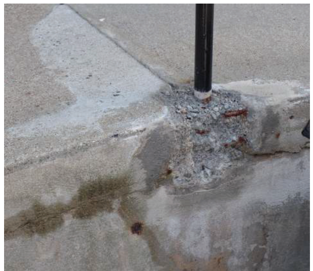
Photo 20: Concrete Damage at Railing Base - Main Campus
