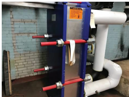
HS Main Building Heat Exchanger
