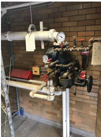
Remote dry alarm valve
