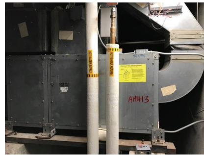
Pool Basement - AHU
