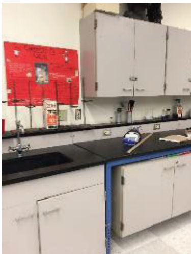
GFCI Receptacles in Science Lab
