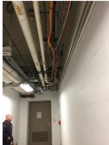
Exposed Data Cabling
