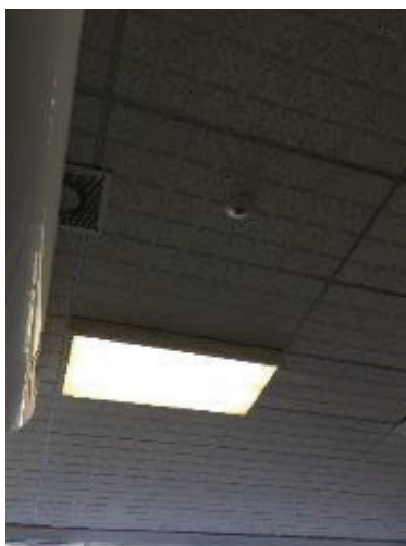
Surface 2'x4' Lighting
