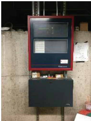
Fire Alarm Control Panel
