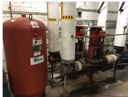
UAB - Hot Water Pumps & Expansion Tank
