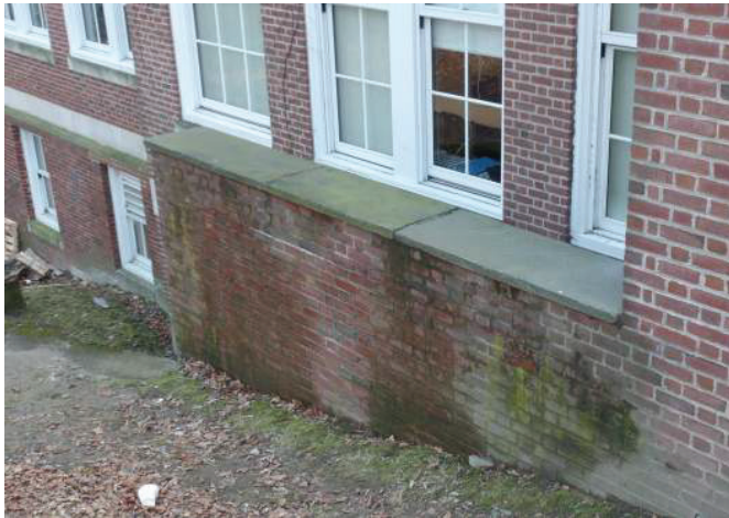
Photo 21: Moisture Damaged Veneer - Main Campus
