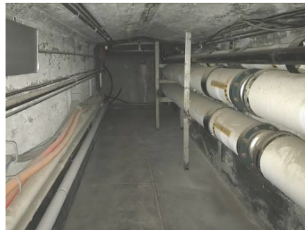
Hot Water Piping in Tunnel
