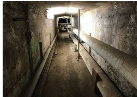
Main HS Building Tunnel – Hot Water Piping
