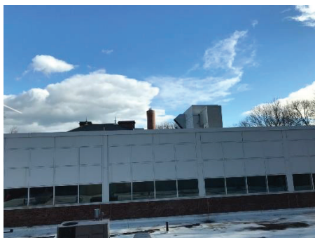
Pool – PoolPak Rooftop AHU
