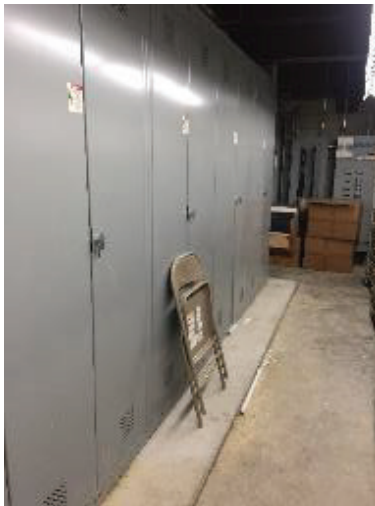
Rear Access to Main Switchgear
