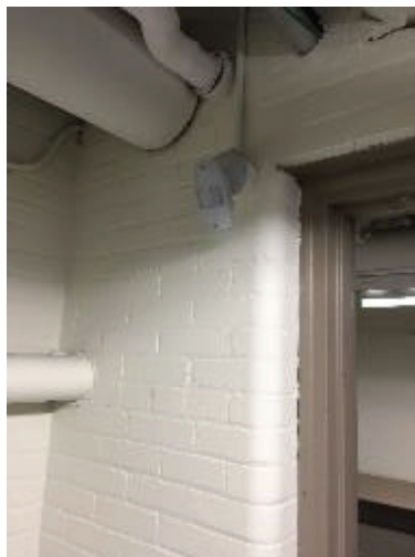
Corridor Occupancy Sensor
