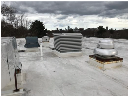
Roof Intake Hood and Exhaust Fan
