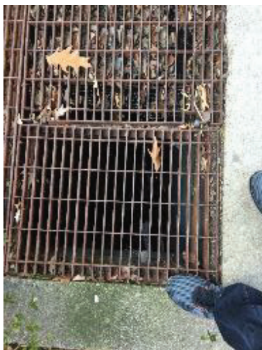
Transformer Vault Grate
