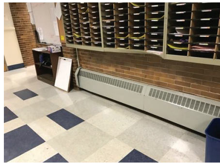
Office area – Fintube radiation
