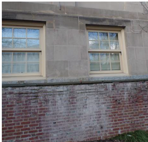
Photo 11: Moisture Damaged Veneer - Main Campus
