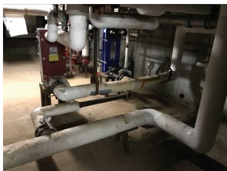
Pool Building – Heat Exchangers
