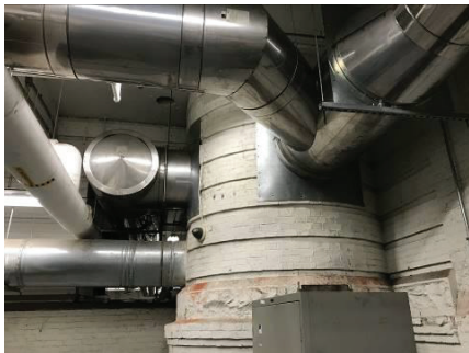
Boiler Breaching
