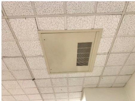
Science Classroom Unit Ventilator
