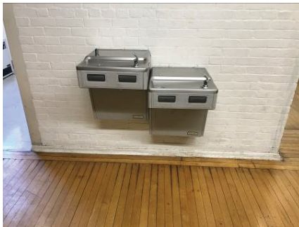
Electric water cooler
