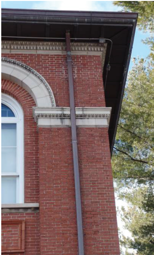
Photo 27: Repair/Repointing of Brick Veneer Needed at Downspout (Moisture Damage) - Unified Arts Building
