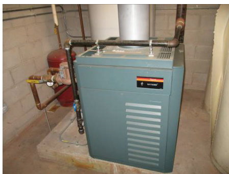
Domestic water heater #2
