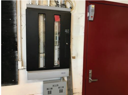
Unified Art Building DDC Control Panels
