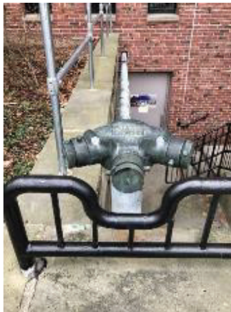
Fire Department Connection Tappan Street
