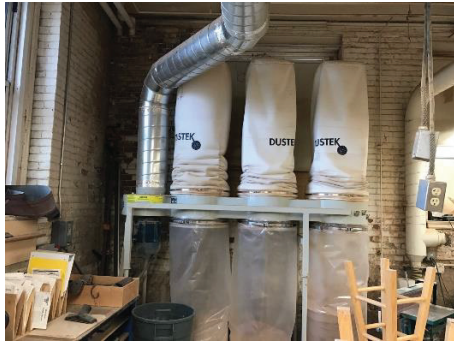
UAB Basement Shop – Dust Collector System
