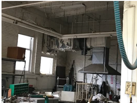
UAB Basement Shop – Canopy Hood Exhaust System
