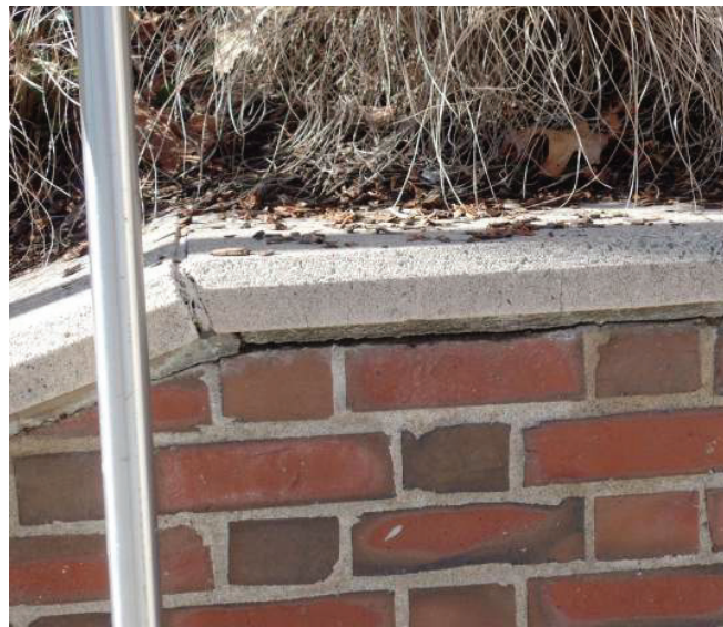
Photo 14: Open Cap Stone Joints at Entry Stair - Main Campus
