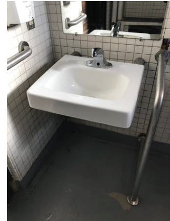
Wall hung lavatory
