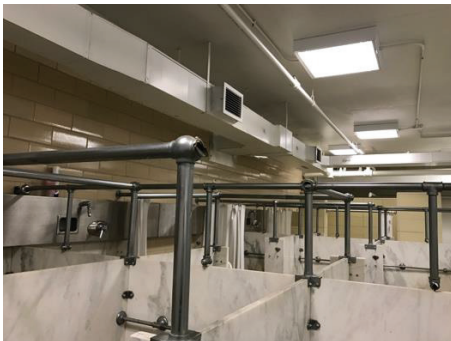
Locker Room Ductwork & Diffusers
