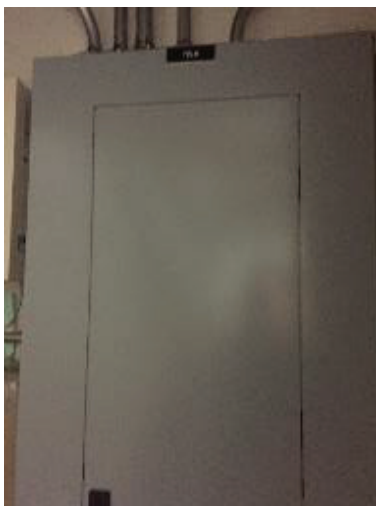
Panel TELB in 2-Hour Rated Closet
