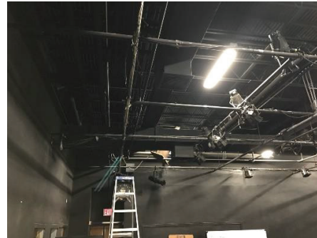
Black Box – Exposed Ductwork
