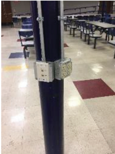
Surface Mounted Receptacles in Cafeteria
