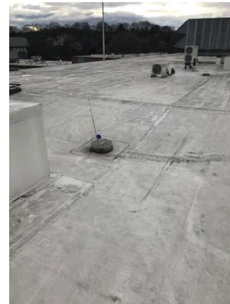
Typical Roof drain
