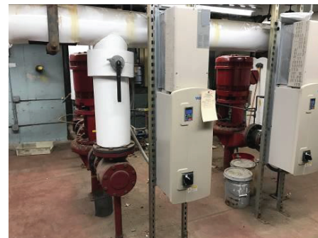
HS Main Building – Hot Water Pumps and VFDs
