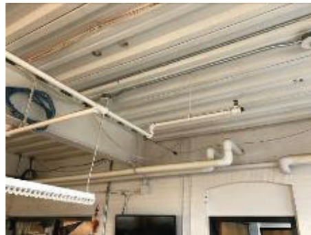
Typical exposed sprinkler piping and upright sprinkler heads
