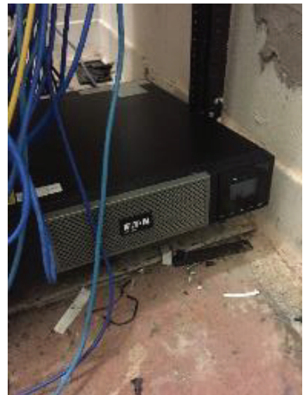
UPS Subject to Damage
