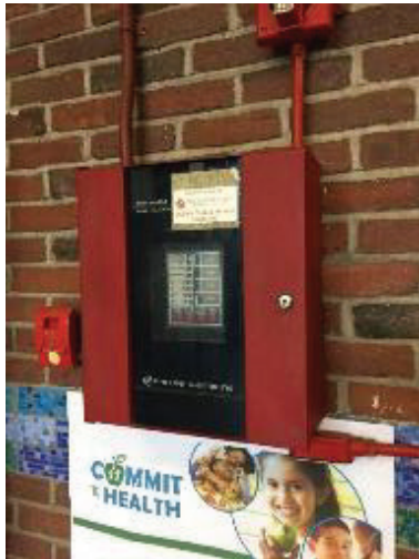
FACP Pool Building
