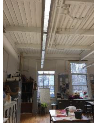
Pendant Direct/Indirect Fixture
