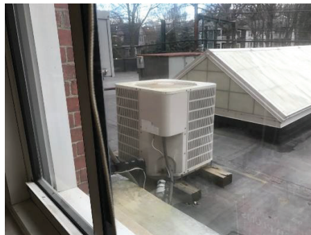
UAB – Roof mounted ACC Unit
