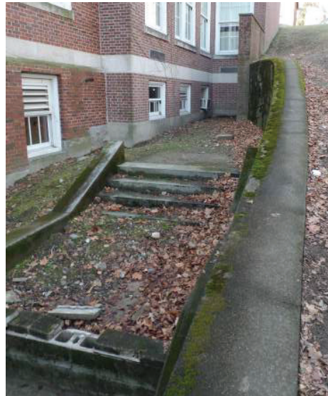
Photo 22: Damaged Site Stairs and Site Walls - Main Campus
