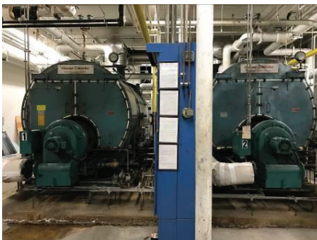
Existing Boilers, B-1 & B-2
