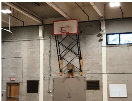
Second Floor Gym – Sidewall Return Registers
