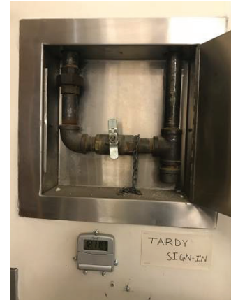
Science room gas shutoff valve
