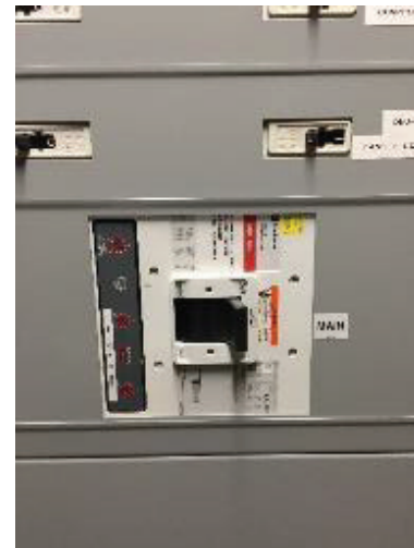
"INDP" Main Circuit Breaker
