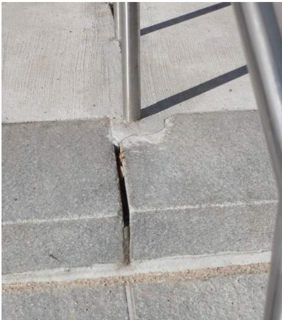
Photo 13: Open Entry Stair Stone Tread - Main Campus
