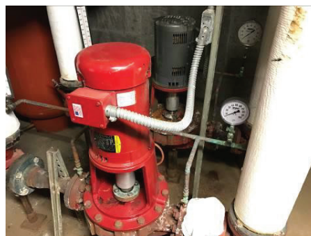
Pool Building – HW Pumps
